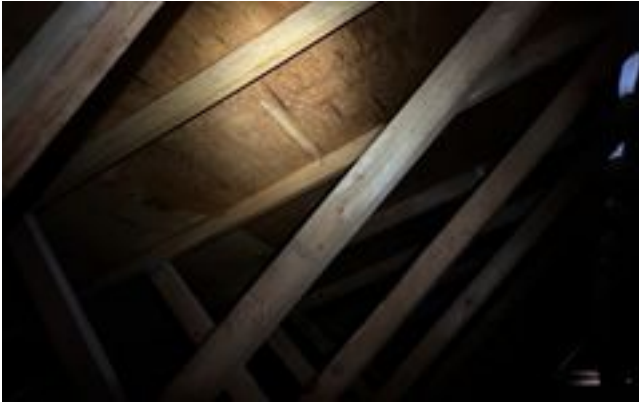
Roof Deck Material – Attic View
