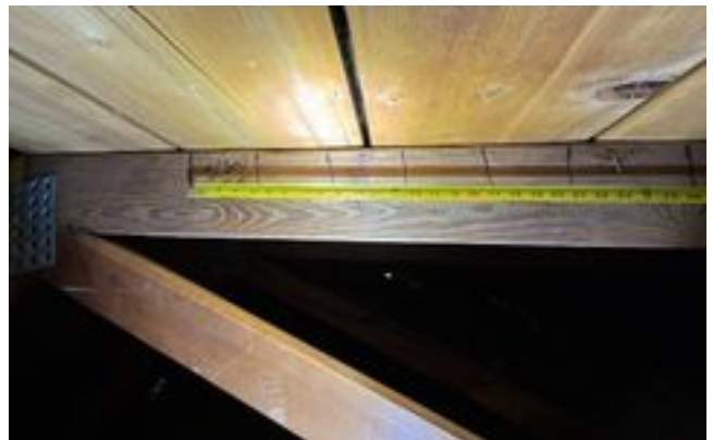
Rafter Bearing on Top Plate
