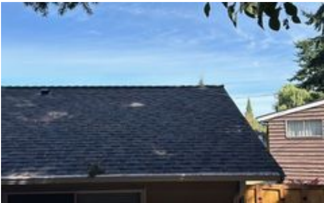
Left Side Roof Slope
