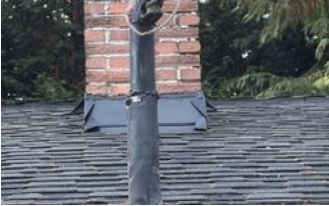
Front Roof Slope
