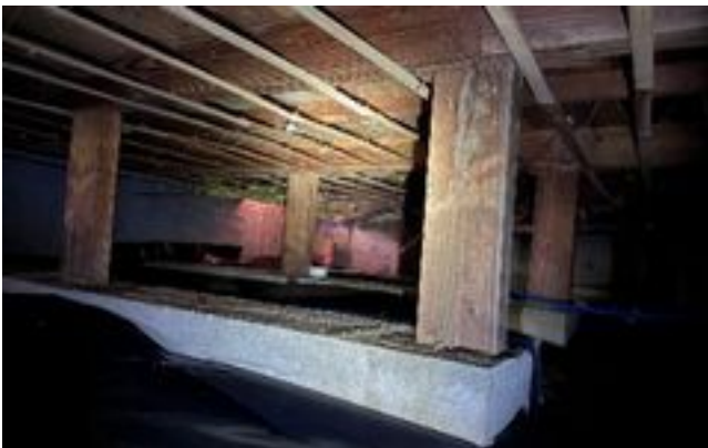
Roof-to-Wall Attachment Area
