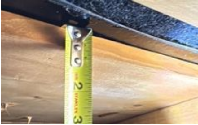
Roof Framing at Wall Connection
