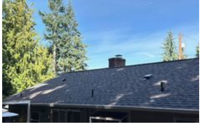
Rear Roof Slope
