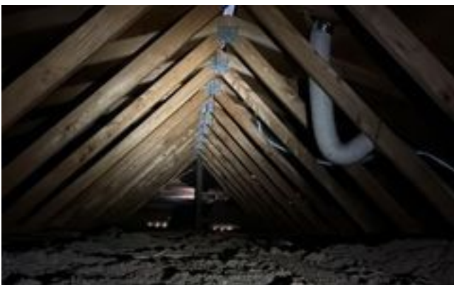
Attic Overview – Roof Framing
