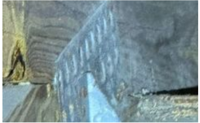
Roof-to-Wall Attachment Detail
