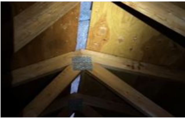
Roof Framing at Ridge Connection
