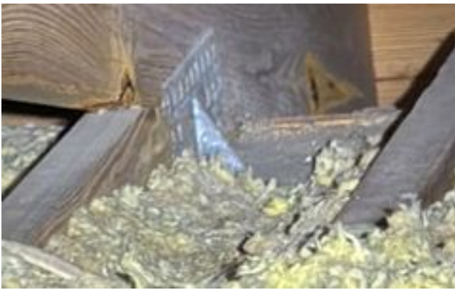
Roof-to-Wall Connection Detail
