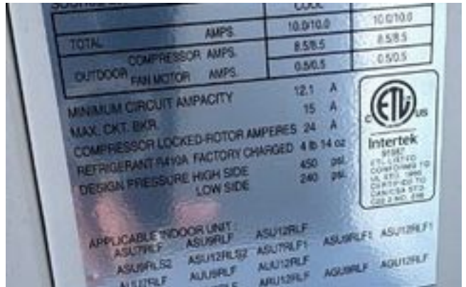
Manufacturer data plate for outdoor unit
