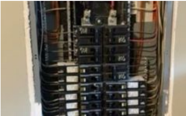
Main electrical service panel with cover removed
