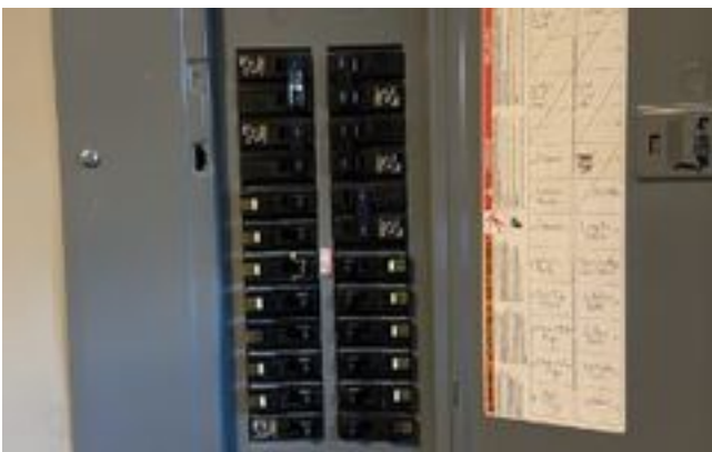
Main electrical service panel open
