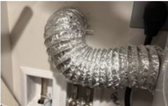
Laundry area vent duct and water connections.
