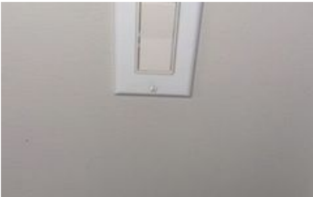
Loose switch plate
