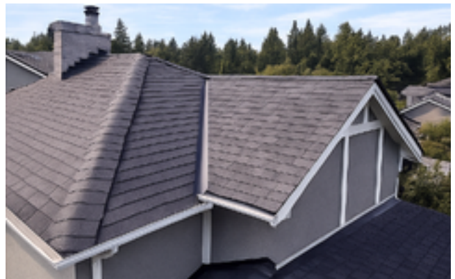
Rear roof slopes, ridge line, and intersecting gables
