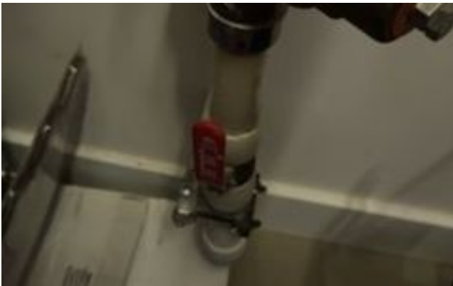
Cold water shutoff valve for water heater
