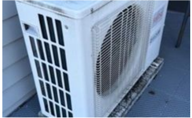
Outdoor Fujitsu condenser mounted on elevated pad
